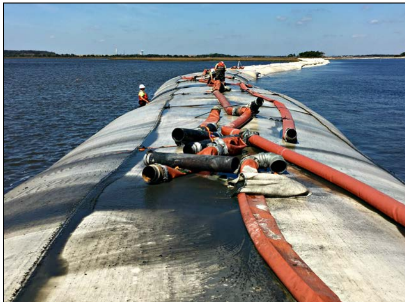
Figure 10. Working around the tides.
