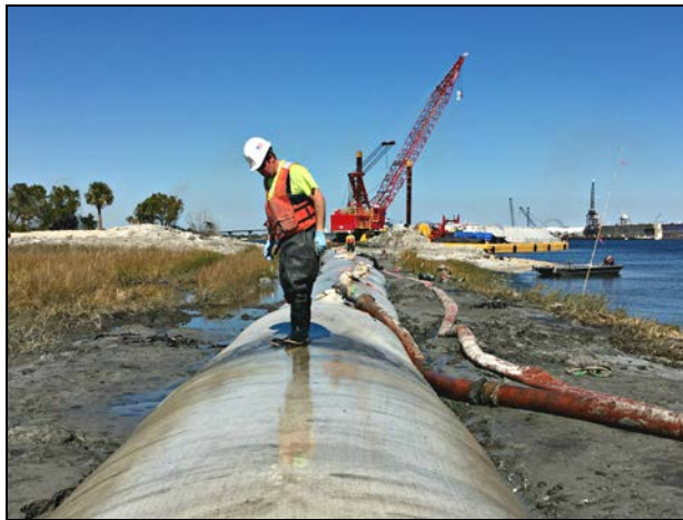
Figure 6. Land side geotextile tubes installed over compacted sand.
