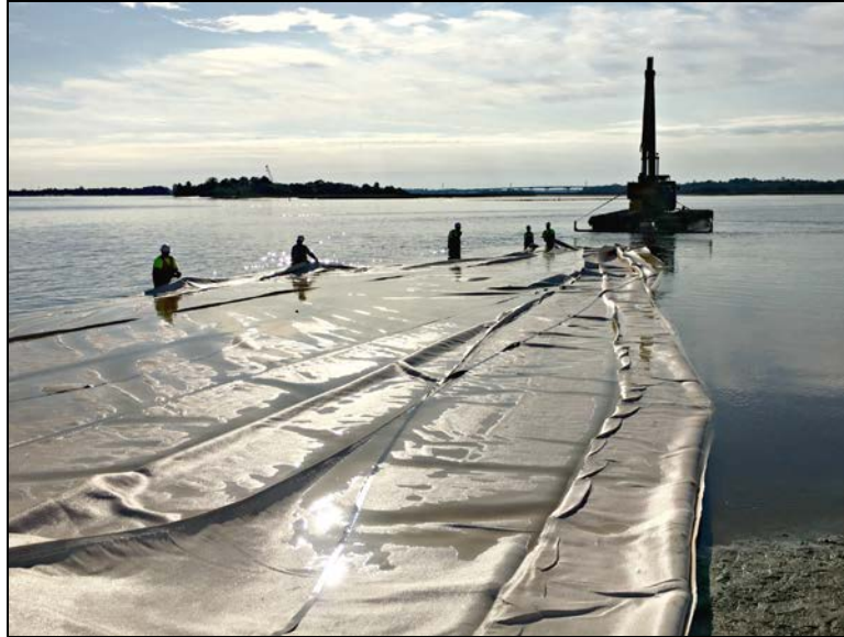
Figure 7. Deploying scour apron with the marsh excavator.
