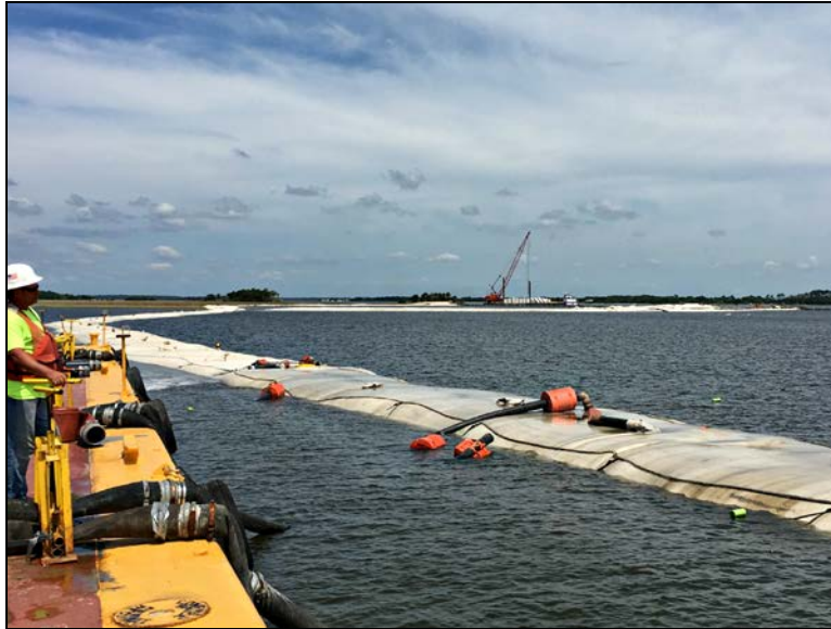
Figure 11. Filling geotextile tubes in the water.
