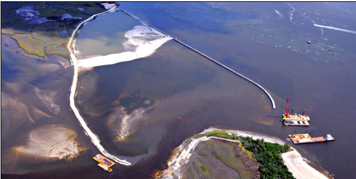
Figure 2. Aerial view of construction of the training wall, including the geotextile tube alignment and installation of precast concrete units.
