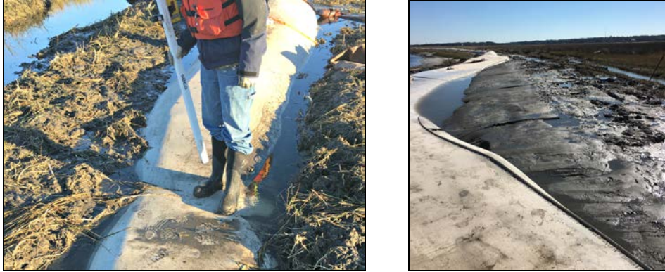
Figures 4 and 5. Filled geotextile tubes, sinking in the marshlands.
