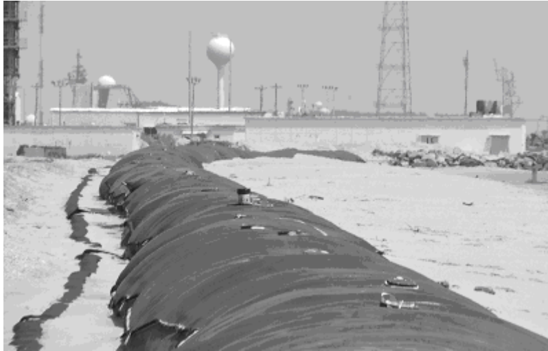
Figure 13 – Filled tubes with natural sand deposition on ocean side.
