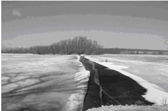
Figure 6 – Tube surrounded by ice
