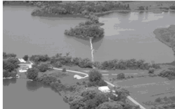
Figure 7 – Aerial view of geotextile tube breakwater
