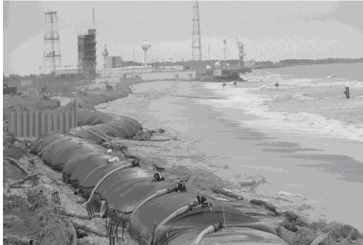
Figure 12 – Geotextile tubes shaped around existing structures.
