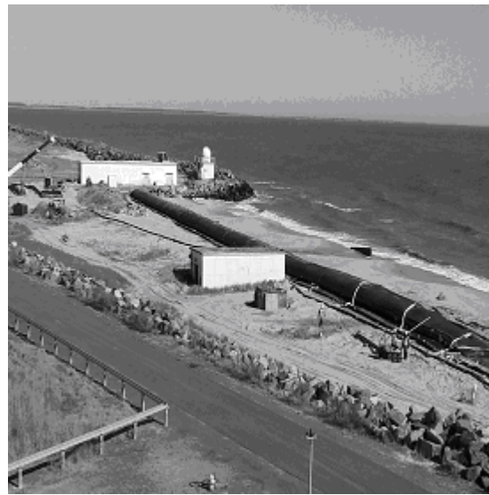
Figure 11- Initial filling at northern end of project site
