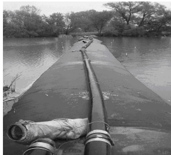
Figure 5 – Final tube fill height
