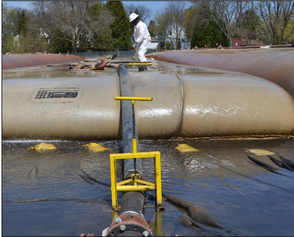
Figure 7. Dewatering Geotextile Tube
