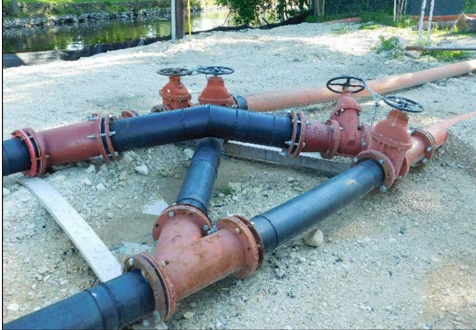
Figure 5. Dredge Slurry Pipeline Flow Control Valves
