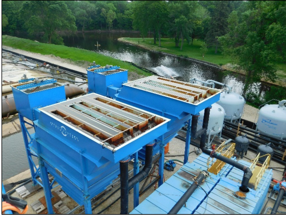
Figure 9. Inclined plate clarifiers
