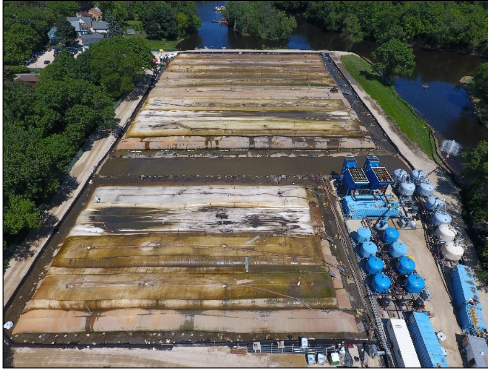
Figure 8. Aerial view of stacked tubes in the SPA
